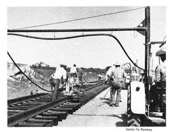
Metal arm and hose line — for welding steel rails — make appropriate frame for track laying operation.
